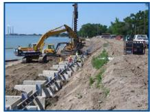
gabions. Geotextile fabric was installed under the concrete and rock for protection of the shoreline. The temporary roadway was removed upon completion of work.
