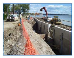
job site. The panels were lifted into place between the galvanized soldier pile, which were placed on 8 ft. centers. The piling was installed into augured excavation approximately 3-4 feet into bedrock and filled with concrete.
